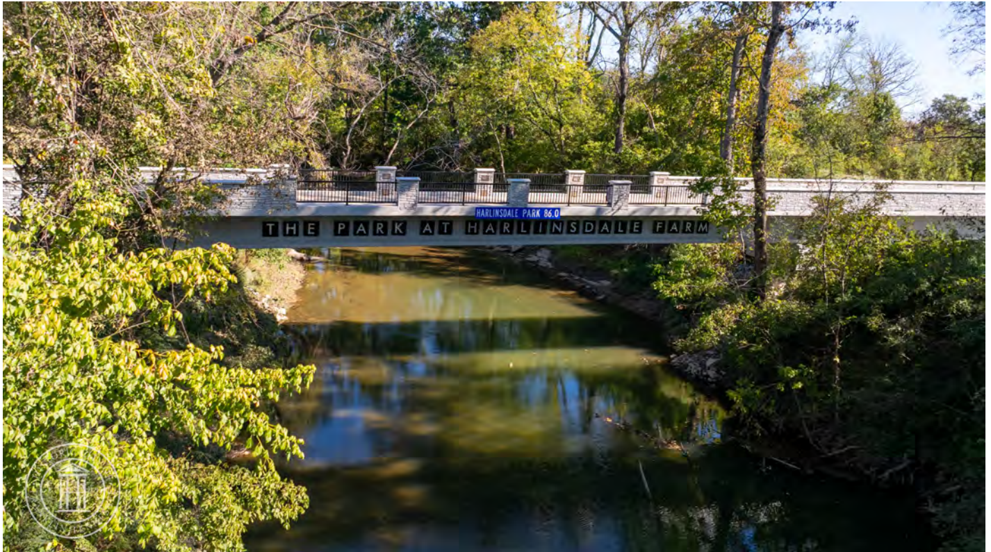
Opening of Pedestrian Bridge at The Park at Harlinsdale Farm
