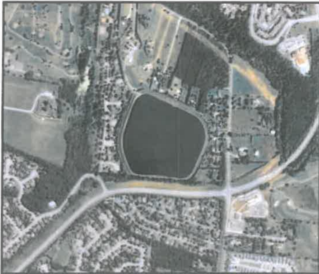
Photo of Franklin Raw Water Reversal provided by Google Earth
