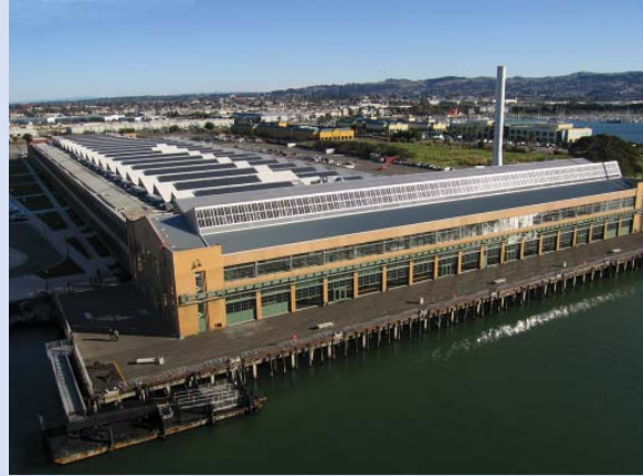
A huge array of photovoltaic solar panels was installed on the south exposure of the monitor roofs in a manner not readily visible by the public. These panels contribute greatly to the energy efficiency of the building. (Kite aerial photo: Michael Layefsky, Great Heights Photography)
