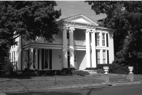
Vaughn/Longino House, Downtown Historic District, both a Local and National Register Historic District.
