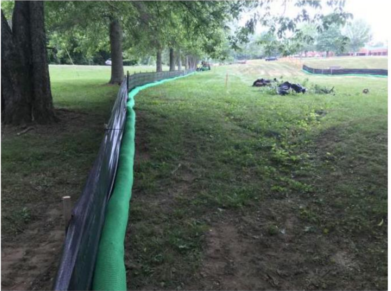
Silt fence installed adjacent to Henpeck LN
