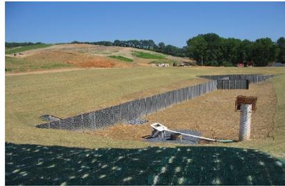
Dewatering devices are required to allow the water to slowly drain down to the permanent wet pool level over a 72-hr dewatering period. Two recommended methods by TDEC are either using a surface skimmer or a perforated riser pipe attached to the principal spillway.
